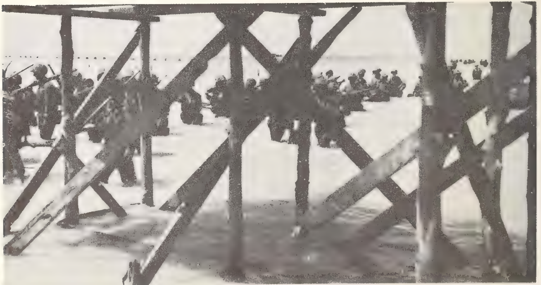
REINFORCEMENTS, seen through the framework of a Japanese pier, wade ashore at Betio. (USMC 63515)
